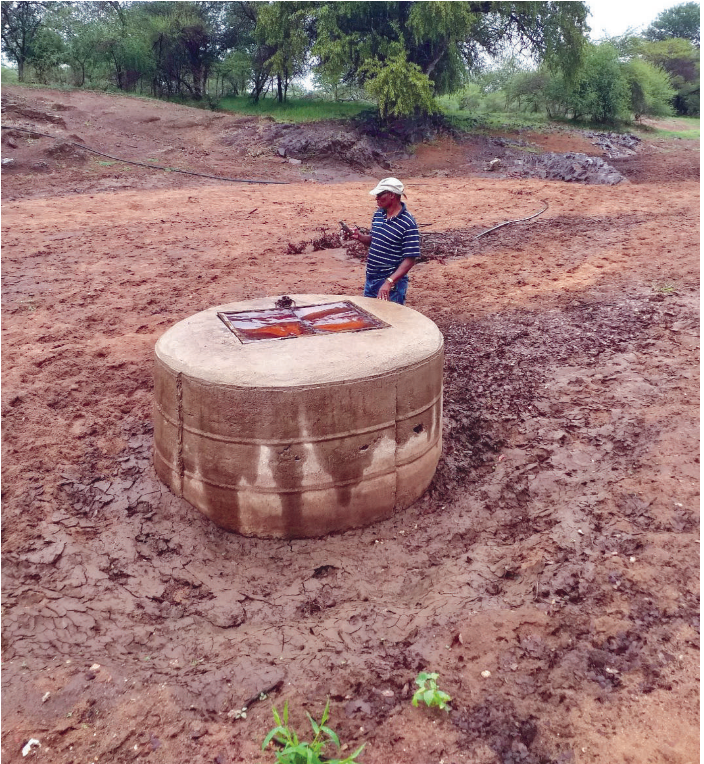
Sand storage tank constructed on the tributary of Motloutse River, Botswana, to collect water flowing through the sand (photo: G. Y. Ebrahim).
